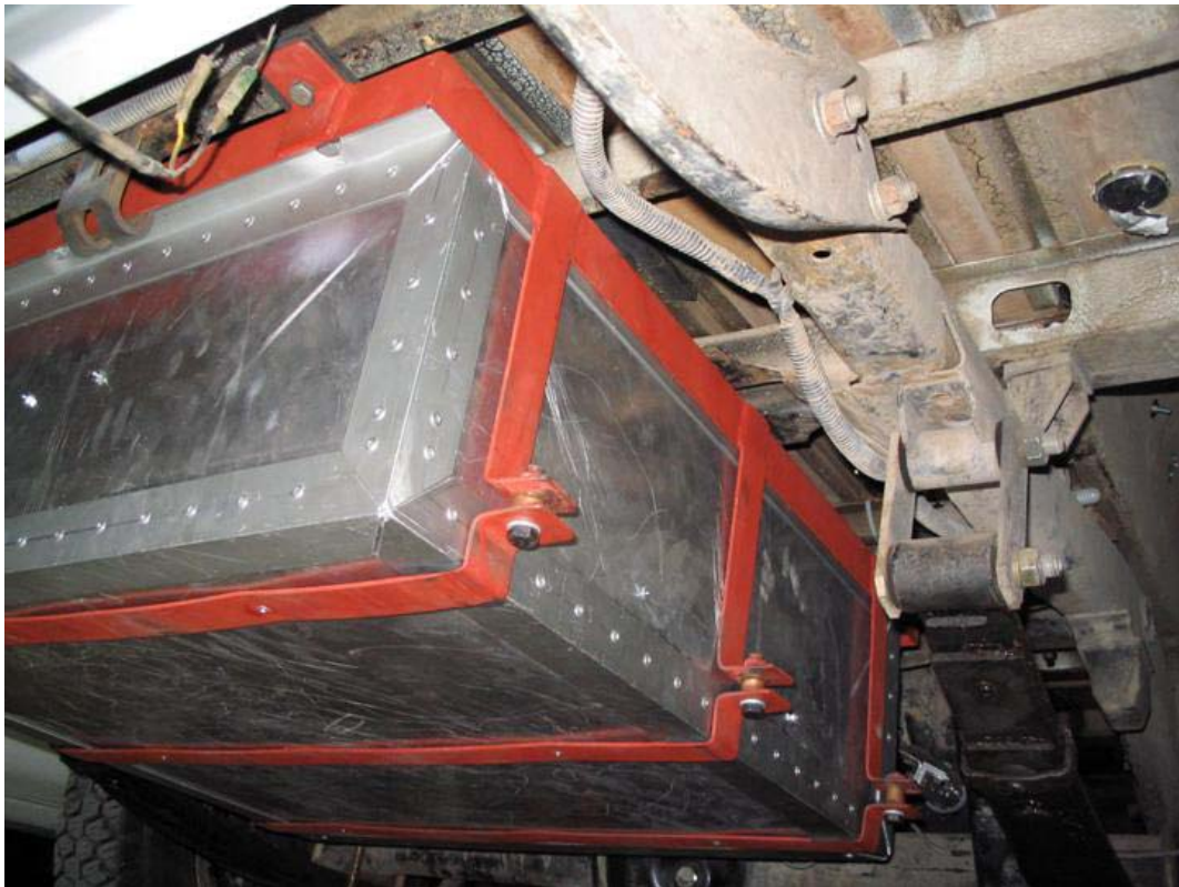
Figure 6: Ultra capacitor bank at the rear, under the floor.
